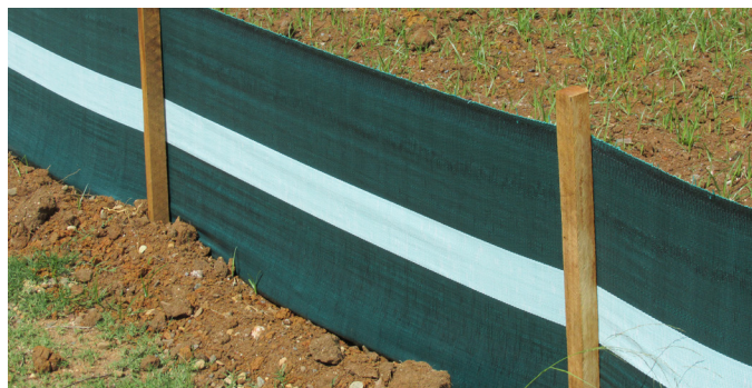
Typical sediment fence. (Source: Healthy Land and Water)
